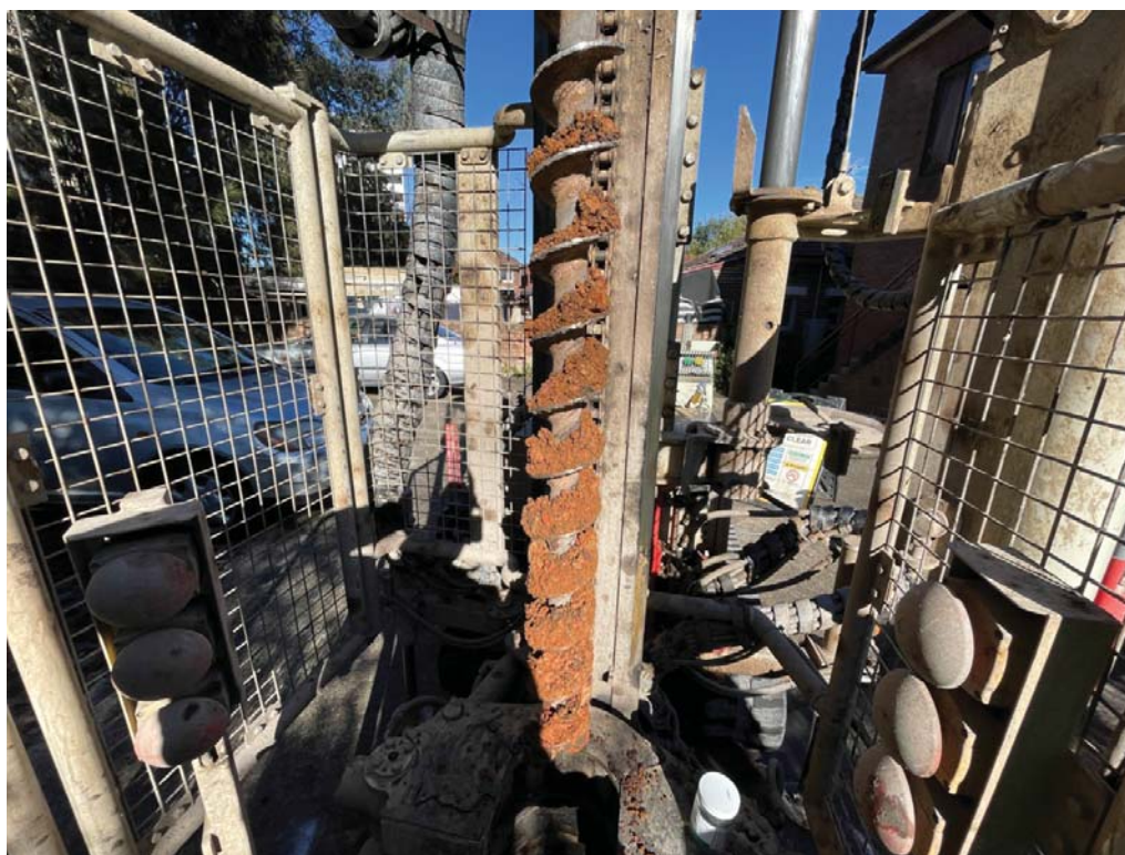
Photograph 2: Drilling at BH204M (17/06/2021).
