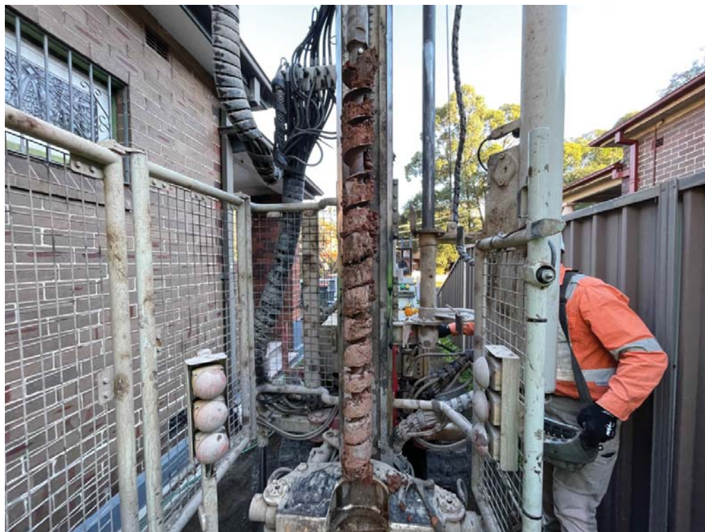
Photograph 1: Drilling at BH201 (17/06/2021).
